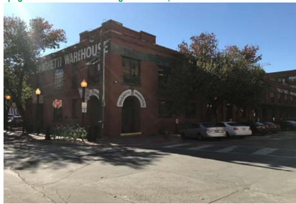
Spaghetti Warehouse Building— West End, Dallas TX
